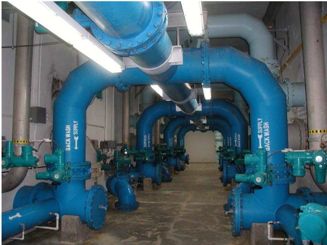
Figure 6-2: Pipe Gallery at South Plant
