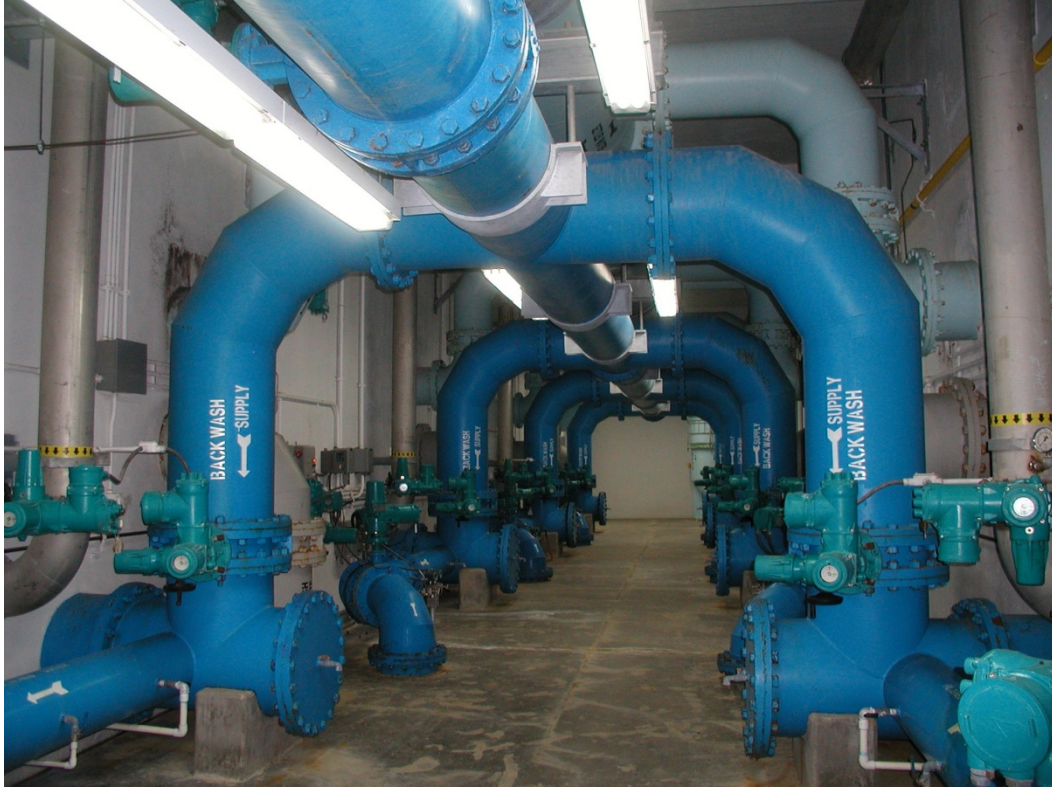
Figure 6-3: Pipe Gallery at South Plant
