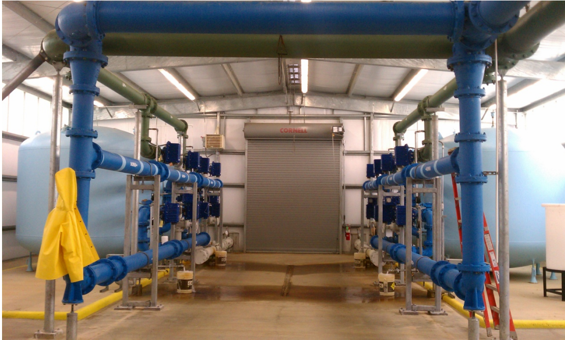
Figure 6-2: Pressure Filters at Well No. 24
