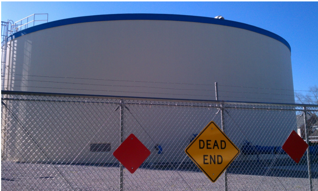
Figure 6-4: Fabacher Field Ground Storage Tank
