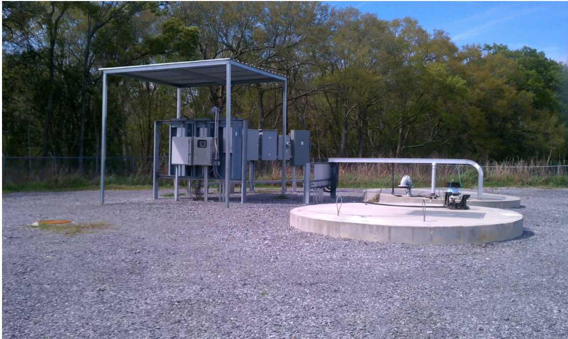
Figure 7-6: Verot School Road Wastewater Lift Station Facility
