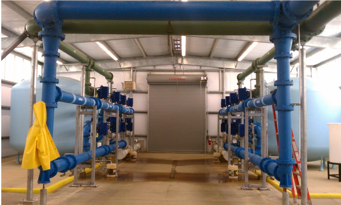
Figure 6-2: Pressure Filters at Well No. 24
