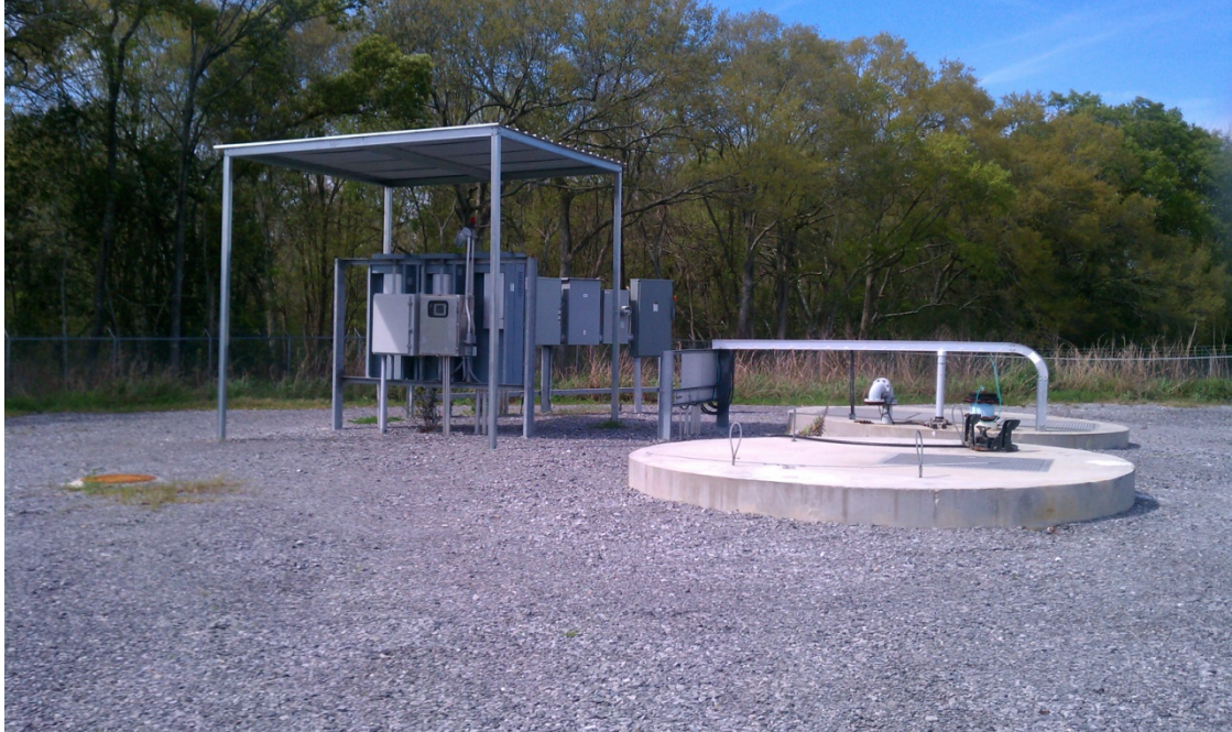
Figure 7-6: Verot School Road Wastewater Lift Station Facility
