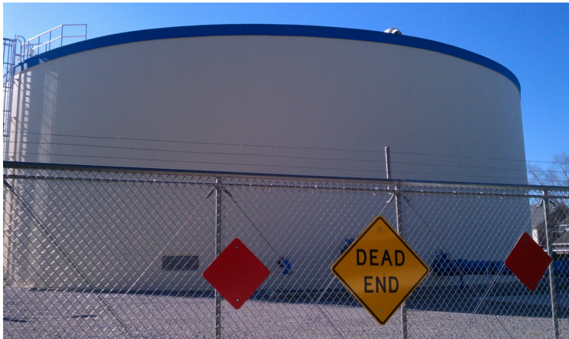
Figure 6-4: Fabacher Field Ground Storage Tank
