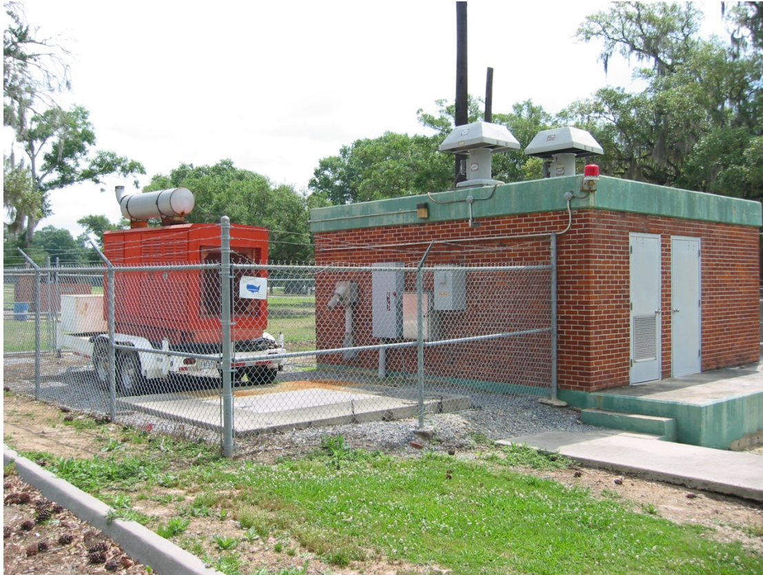
Figure 7-6: Heyman Park Wastewater Lift Station Facility
