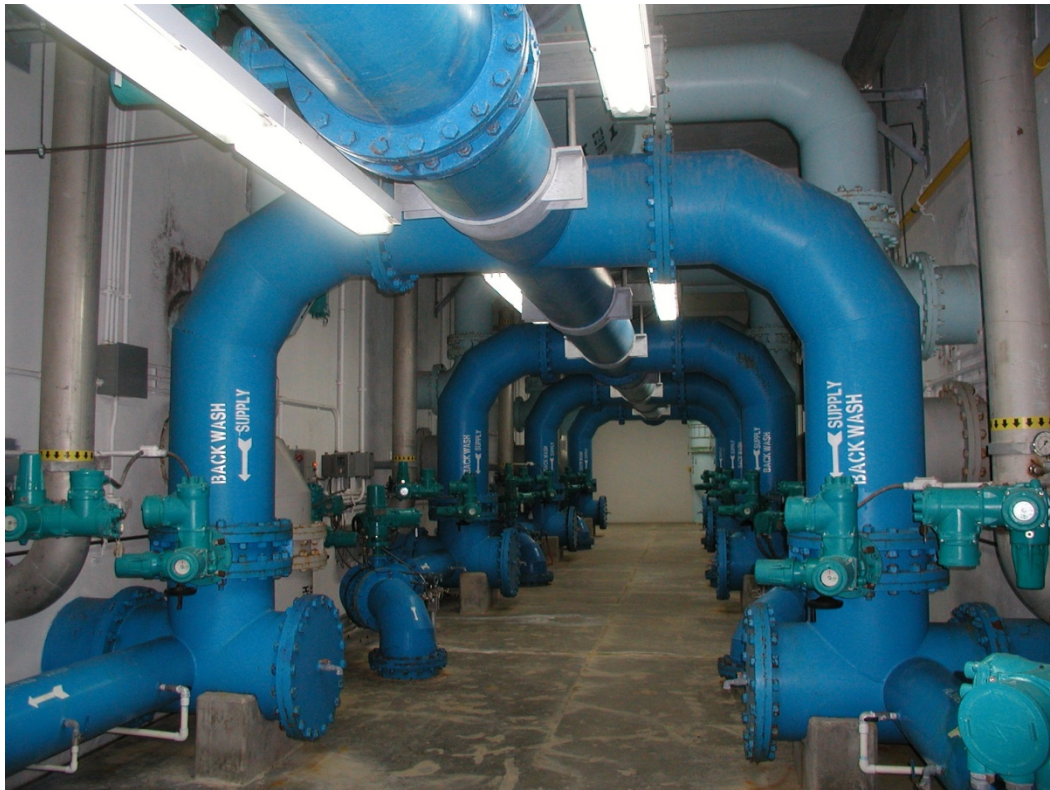
Figure 6-2: Pipe Gallery at South Plant
