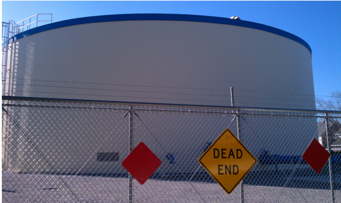
Figure 6-3: Fabacher Field Ground Storage Tank
